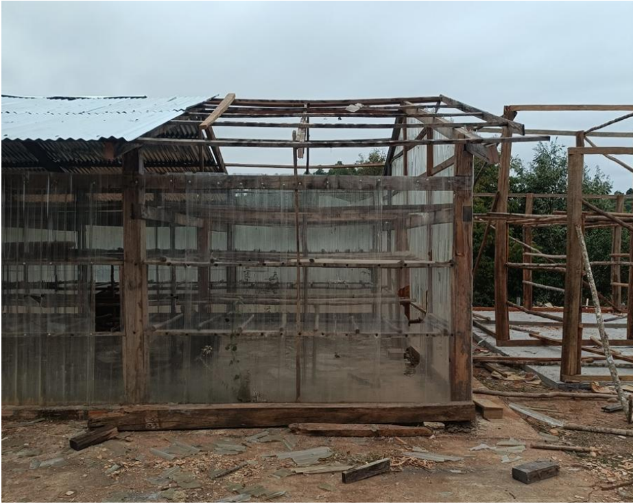
Photo 13. The extended drying area will be roofed by plastic film.
