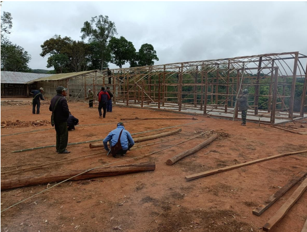
Photo 13. The extended drying area will be roofed by plastic film.
