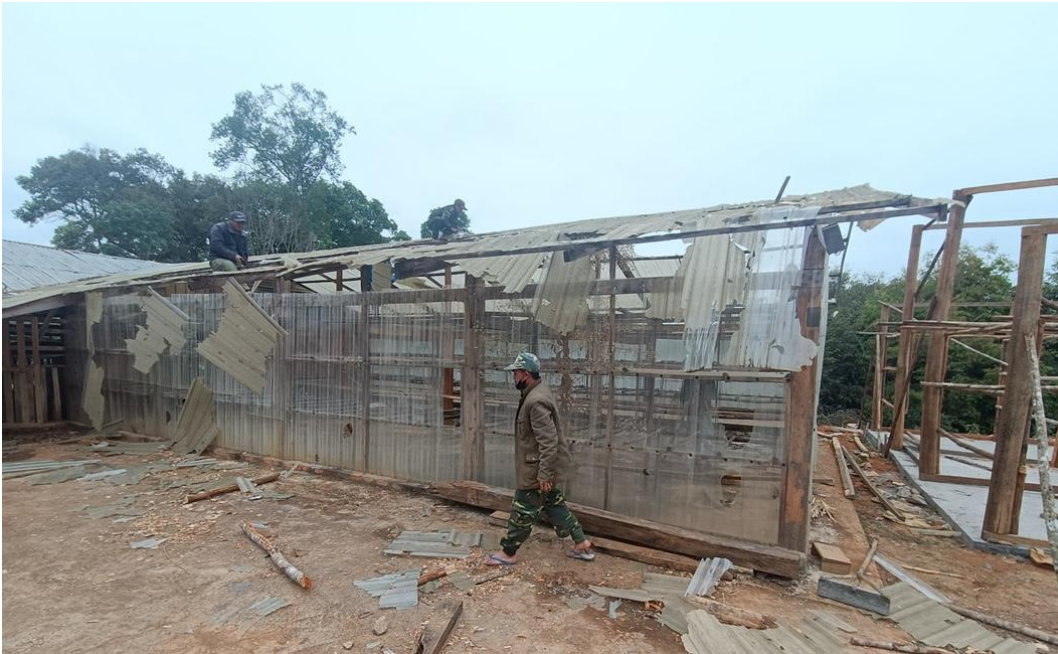
to new zinc roof
