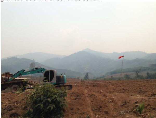
An excavator preparing the field for the next crop of bananas.
